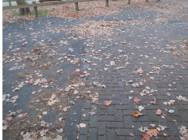
**Figure 13. Permeable Paver Installation in Sanford.**
