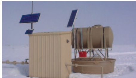
A solar-powered methanol injection pump.
