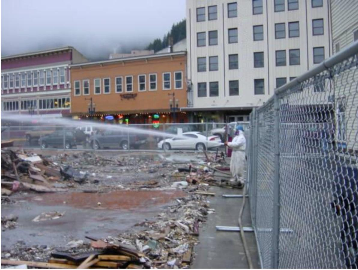
*Figure 5. The surrounding sidewalk functions as a berm at this demolition, (EPA photo courtesy of John Pavitt, Region 10).*
