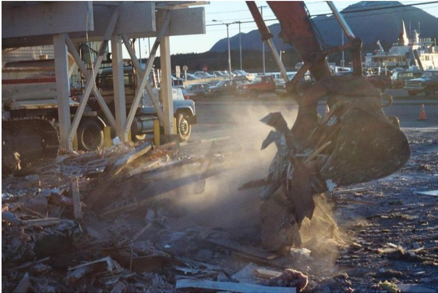
Figure 2. This photo illustrates the practical need for adequate wetting of asbestos contaminated materials. Dust containing asbestos is released when ACM are not removed prior to demolition. (EPA Photo courtesy of John Pavitt, Region 10).
