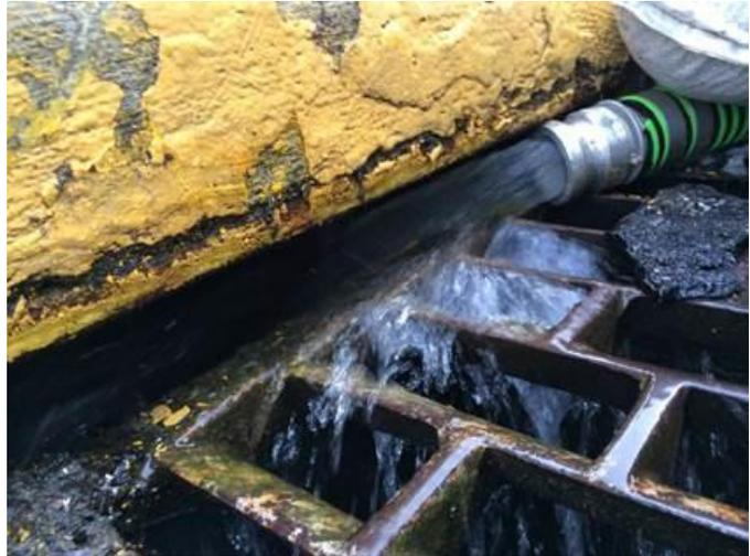
*Figure 10. After filtration and testing of demolition water showed the water met effluent standards, it was released into the stormwater drain adjacent to the demolition project. Photo courtesy of John Pavitt, USEPA Region 10.*
