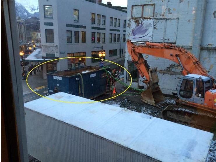
Figure 8. Water from a building demolition drained into the basement and was pumped to this tank (circled in picture) for settling before filtration to remove asbestos and other pollutants. Photo courtesy of John Pavitt, US EPA Region 10.
