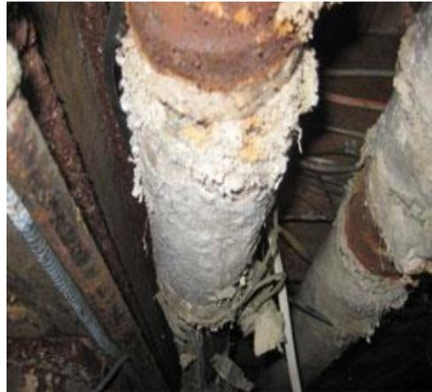
*Figure 14. Pipe wrap is frequently hidden and may be difficult to find. Special wetting agents may be needed for pipe wrap.*
