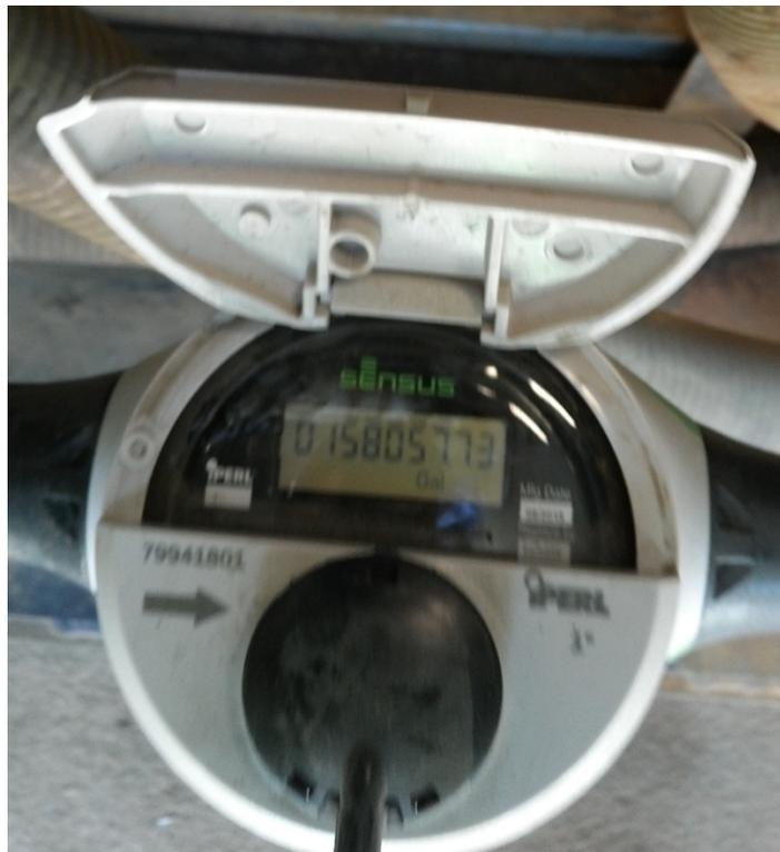
Picture 8: Groundwater Pumping Meter
