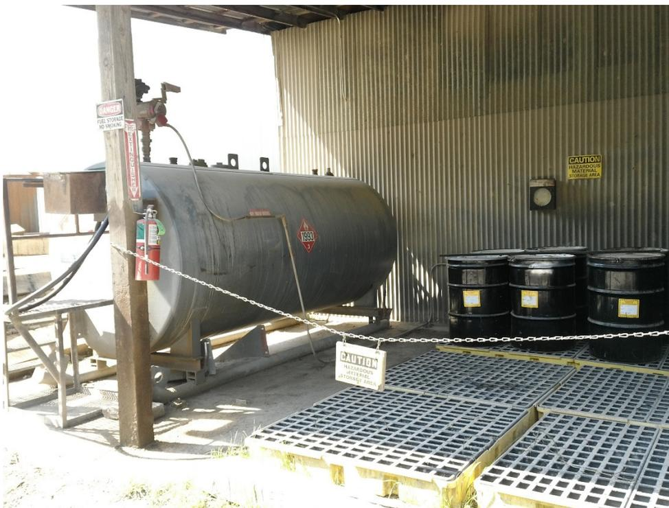
Picture 6: Diesel Fuel Tank w/ containment and Hazardous Waste Storage Area
