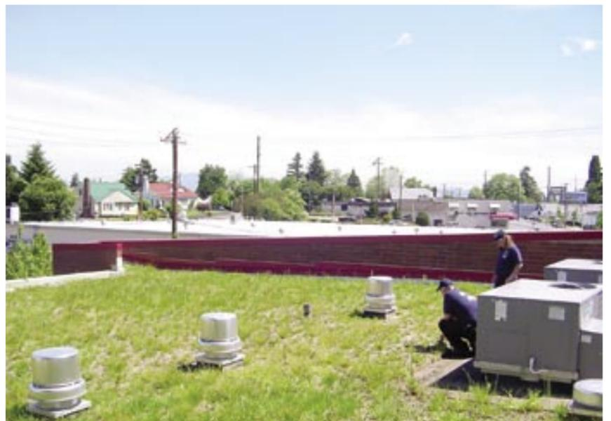
Ecoroofs such as this one at a NE Portland Fire Station are being used with greater frequency as a way to reduce the impervious surface associated with development. Most ecoroofs can absorb close to 100% of the rain that falls on them, significantly lessening the stormwater impacts associated with a traditional roof. Ecoroofs can also reduce heating and cooling costs.
