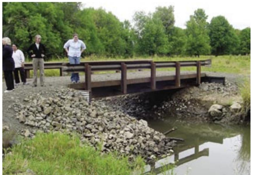
The culvert in the left photo was replaced with a bridge that allows for full fish passage and creates more natural stream conditions that will help maintain lower temperatures, and decrease sedimentation and erosion. Bridges such as this often provide the best long term solution to fish passage problems.
