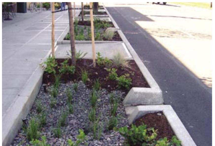
Planting strips like this one in SE Portland in front of the New Seasons Marketplace at 19th and Division may be the wave of the future. Instead of being built to keep road generated stormwater runoff out, they have been built to capture and infiltrate the runoff.
