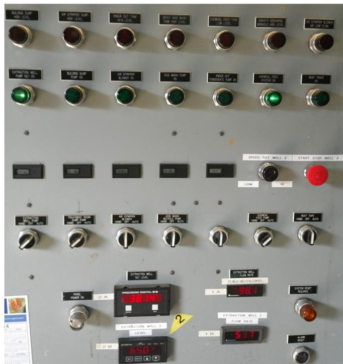
Picture 6: Dual Phase Extraction System Indicators and Flow Meters
