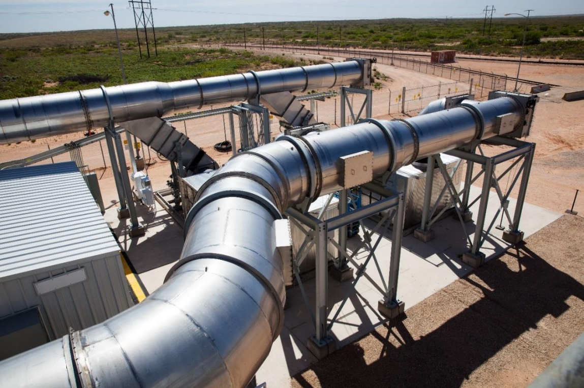
Side view of duct work, filter and fan unit
