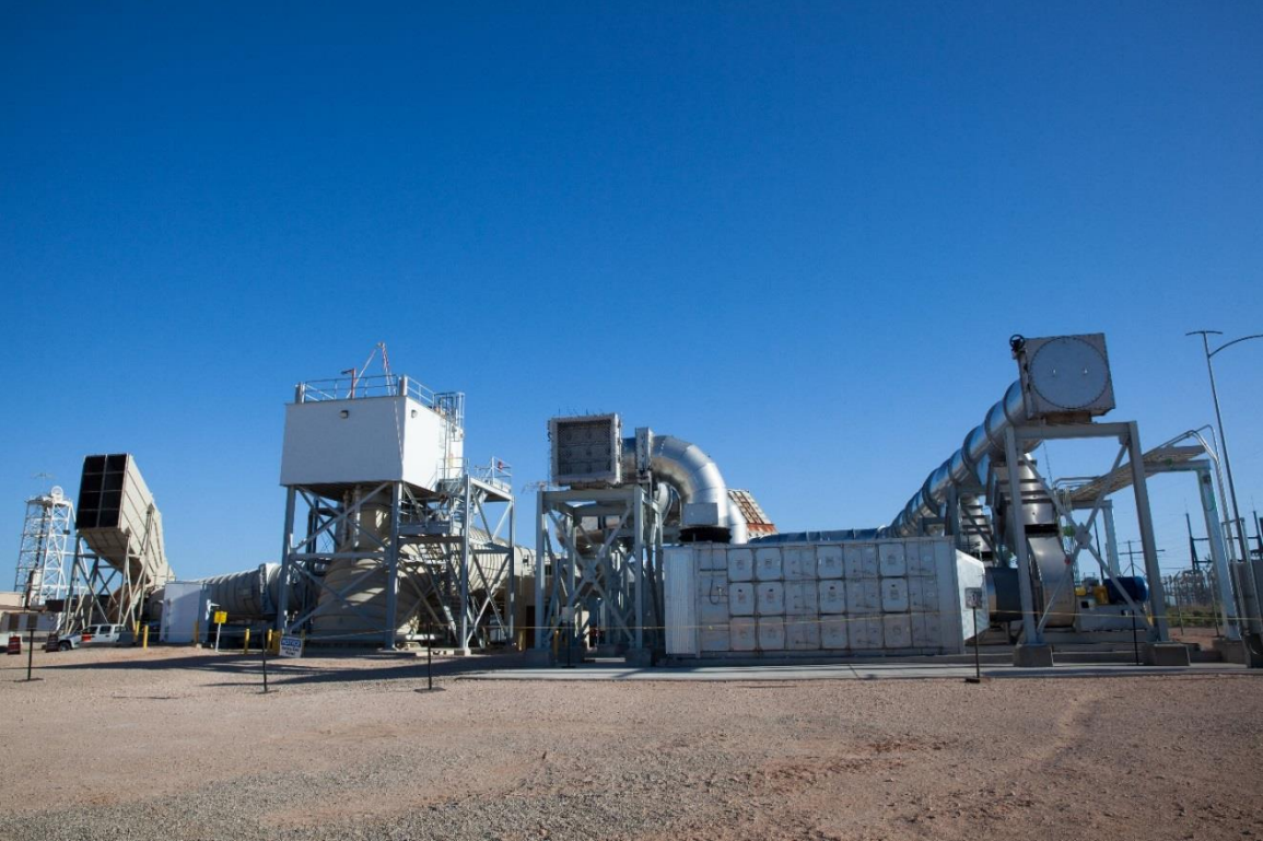
Side view of duct work, filter and fan unit
