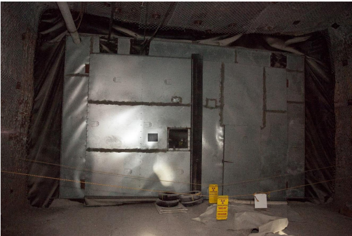
Recently replaced ventilation bulkhead
