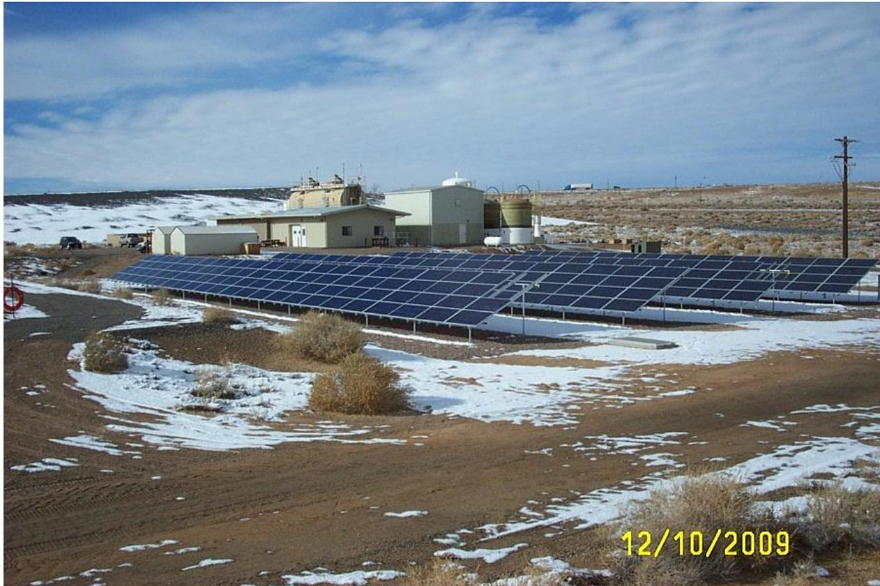
**Figure 9: Solar panels at the Tuba City Disposal Cell**
