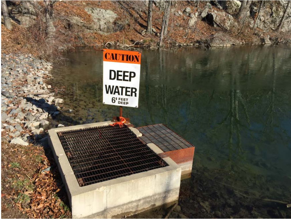
Holding Lagoon (Foster Pond is off to the left of the photograph). Source: site visit, 2016.
