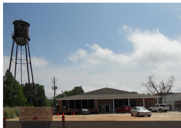
The Shubuta Outreach Family Clinic was one of several properties prioritized for brownfields assessment, cleanup and redevelopment in Clarke County.
