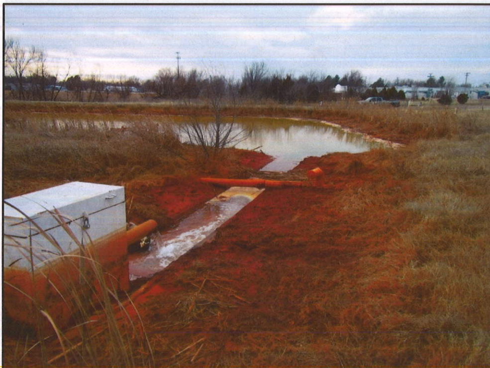
Photo 2: MRPTS Outflow into Oxidation Pond
