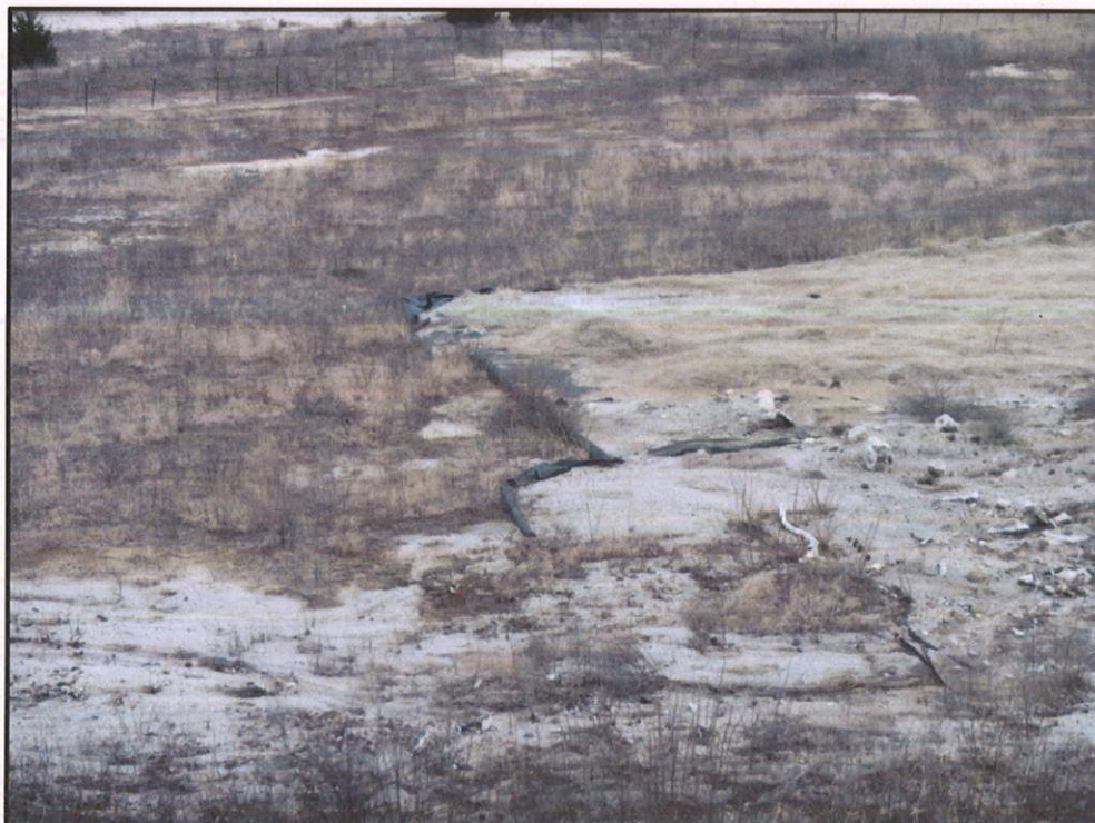
Photo 14: Collapsed Rolled Silt Fence on Northern Side of Central Mill Repository
