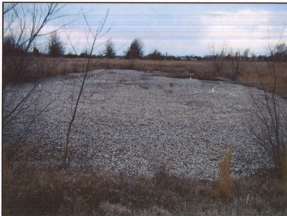
Photo 6: MRPTS Horizontal-flow Limestone Bed
