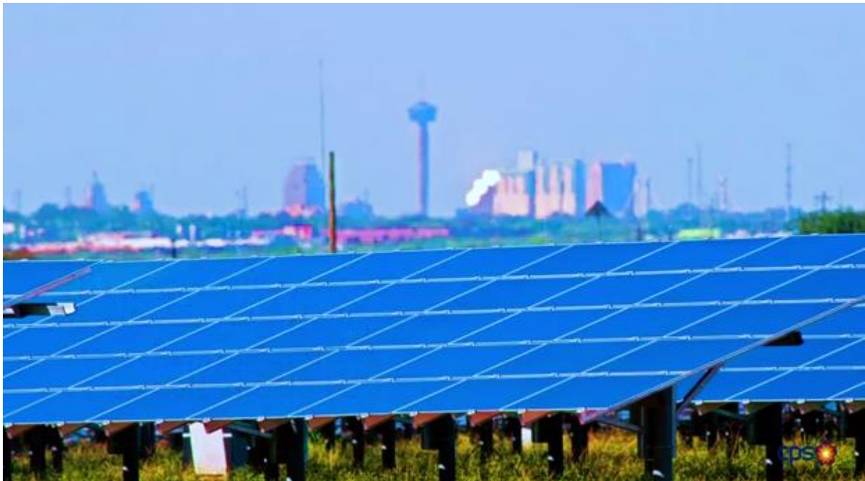
Duke Energy Blue Wing Solar Project supplies electricity to CPS Energy under the terms of a 30-year power purchase agreement.
