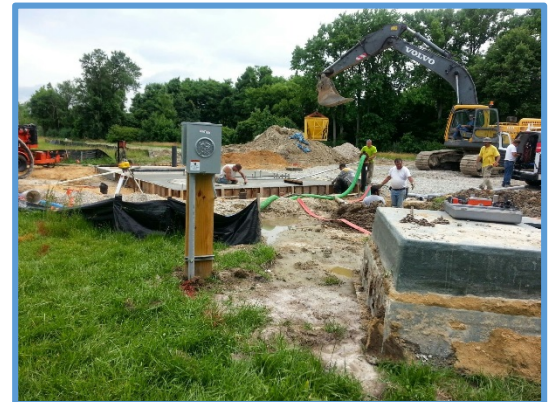
Work to provide mobile home communities with sewer system in Dover.
