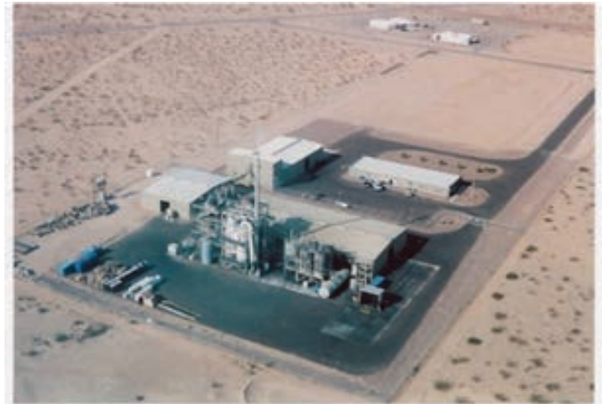
Evoqua Facility in Parker, AZ
