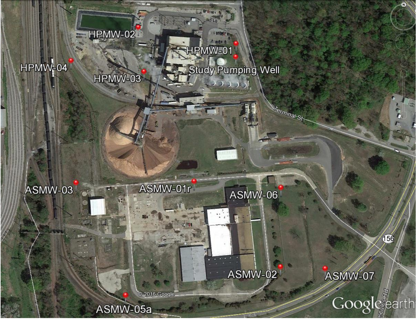
Figure 2: Aerial Map of Firestone Fiber and Dominion Hopewell Power Station with Well Locations
