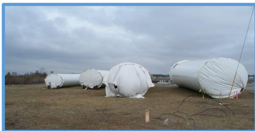
Sections of turbine ready to be installed. Courtesy: City of Crisfield
