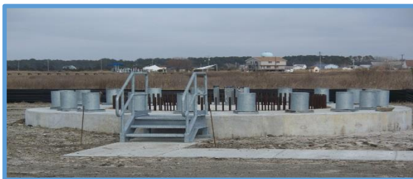
The base of the turbine is prepared.
