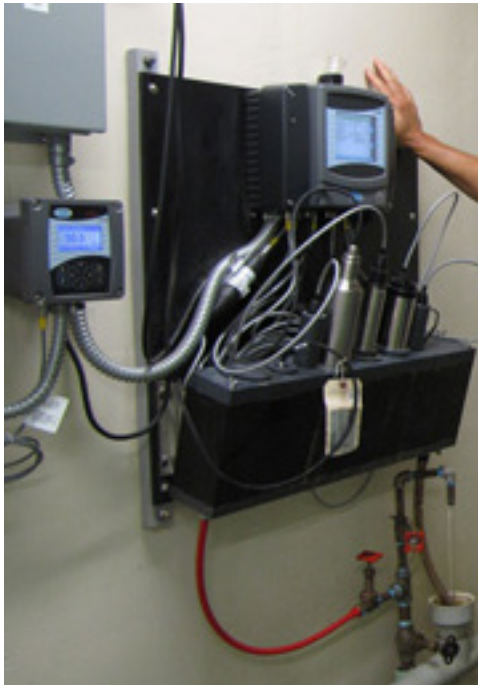
Figure 9-9. RAIN Monitoring Station
