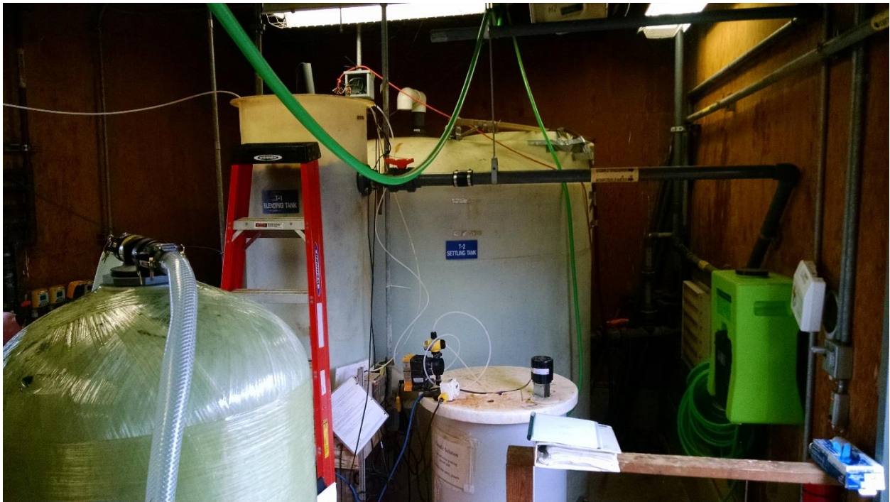
Photo 2. GAC, Soda Ash Reaction Tank (T-1), and Settling Tank (T-2) (December 1, 2015)
