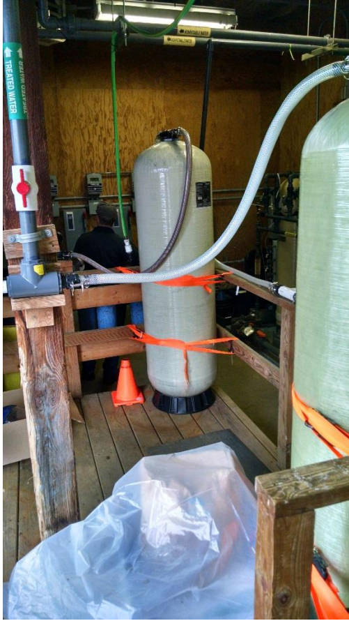
Photo 5. New Fiberglass GAC Canisters (December 1, 2015)
