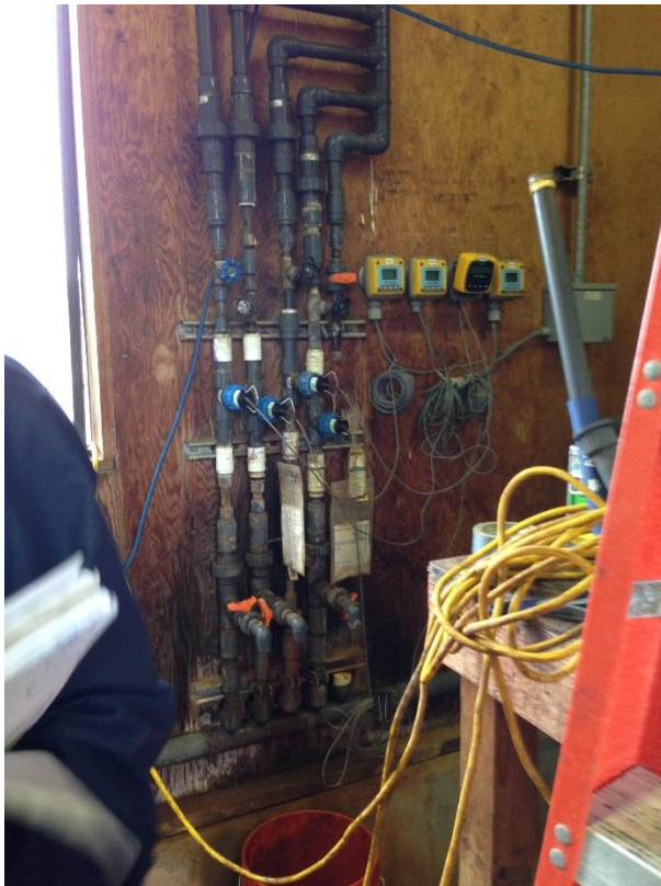
Photo 4. Extraction Well Influent Manifold and Flow Meters (December 1, 2015)
