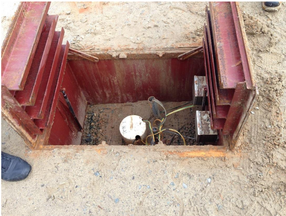
Photo 8. Extraction Well RW-1 Vault (December 1, 2015)
