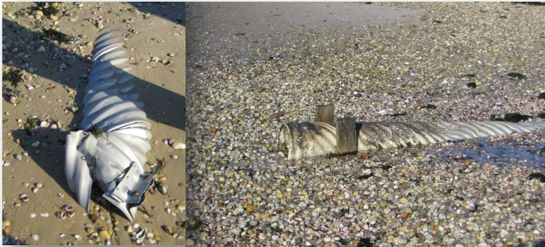
**Figure 8. Culverts/pipes adjacent to Shinnecock Indian Cemetery. Both culverts are clogged, damaged, and in need of repair.**
