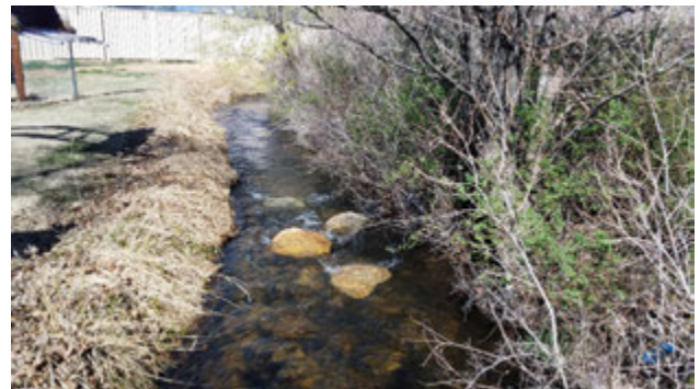
Bishop Paiute Tribe streambank erosion control project. Tribal staff used boulders to slow water flows in the channel to mitigate erosion.
