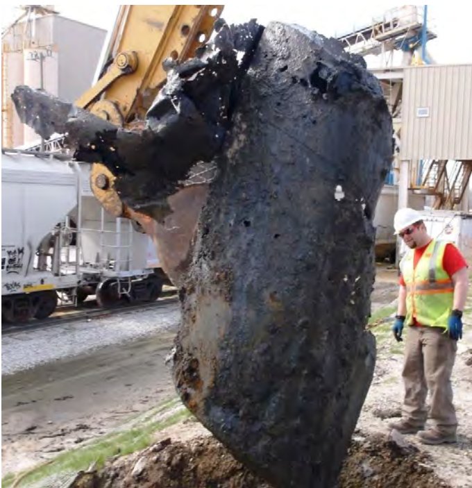
Workers remove a leaky underground storage tank from Illinois Railway property in Wedron. U.S. EPA engineers are looking at several possible sources of well water contamination in the town.
