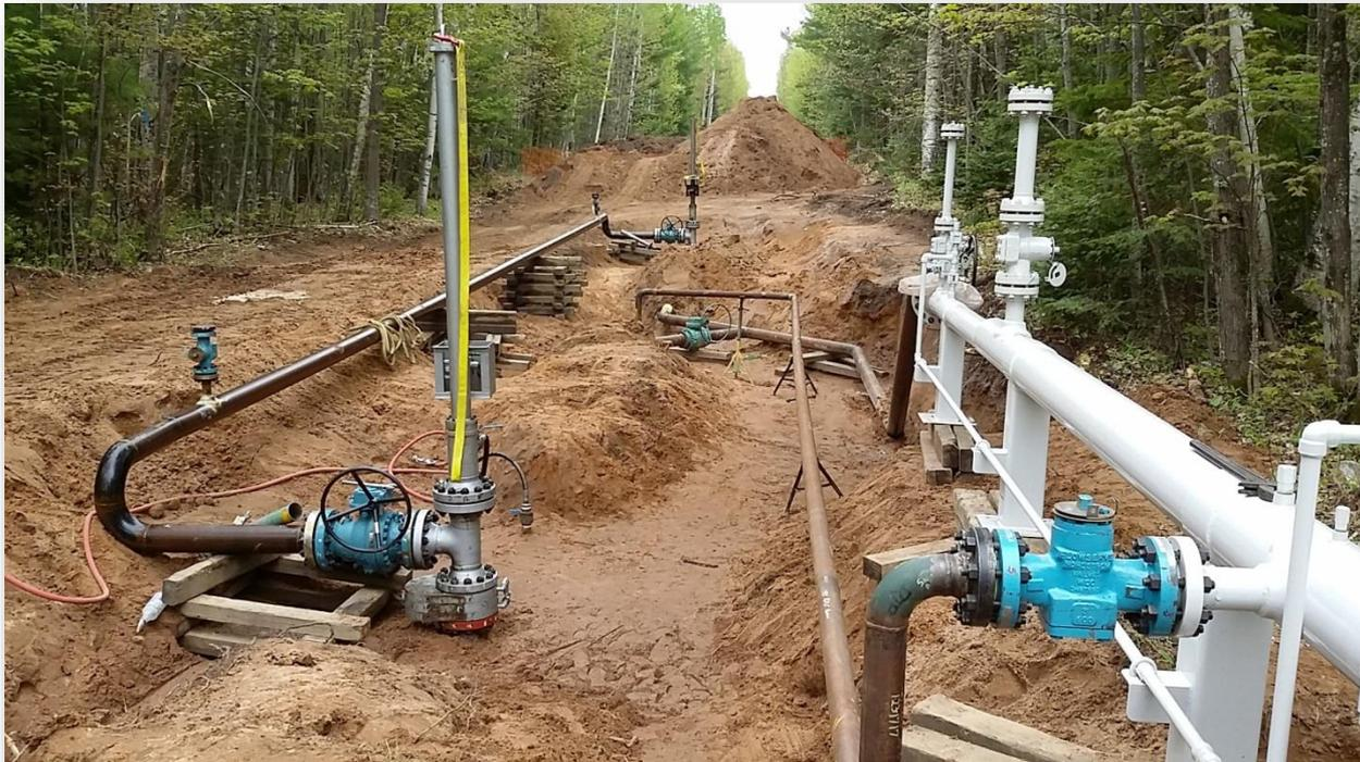
Smaller-diameter pipeline stopple bypass
