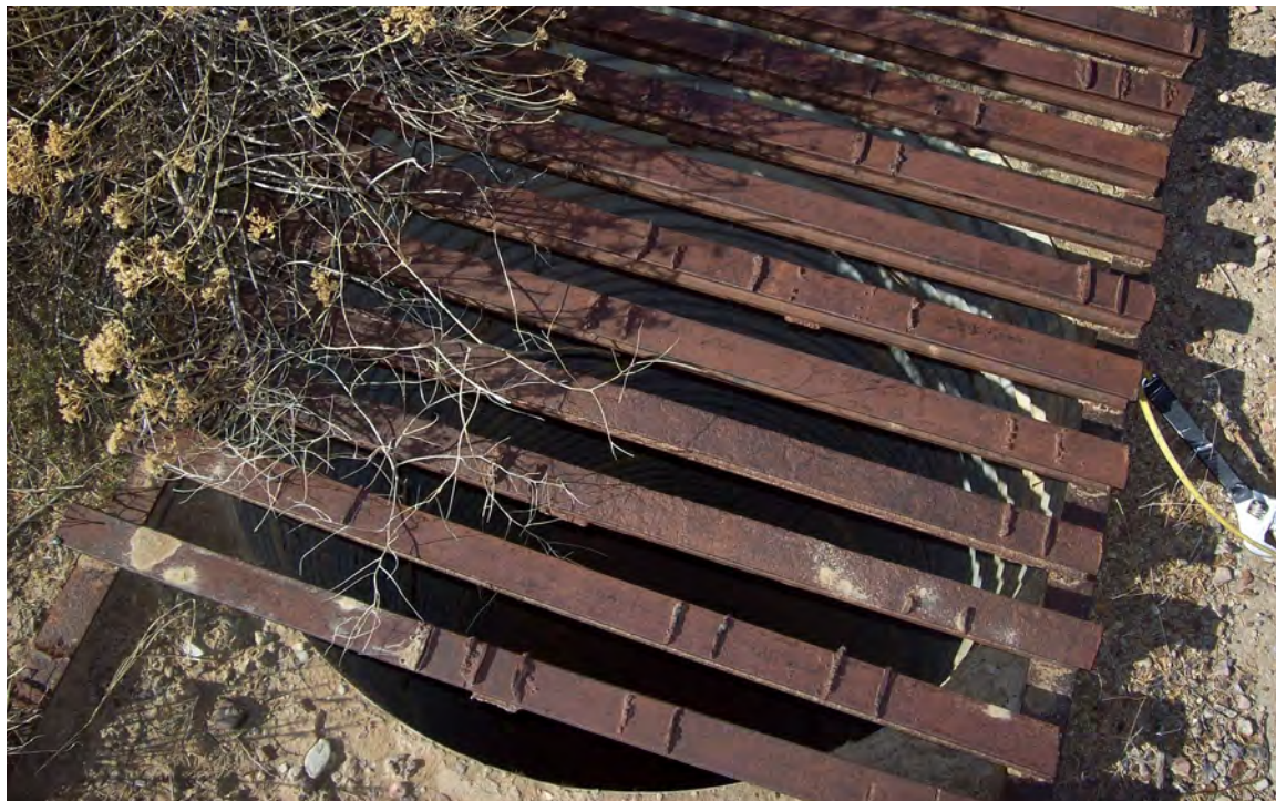
Photo 3-B: Triangle Underground Mine Vent Shaft
