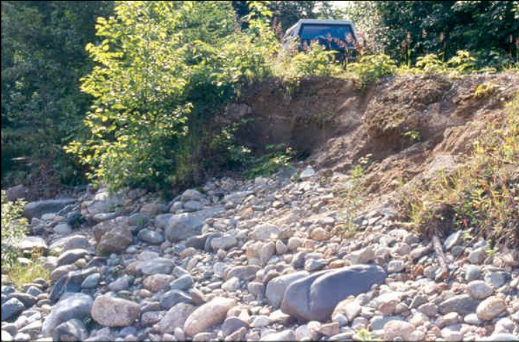
Stream bank erosion along poorly sited road
