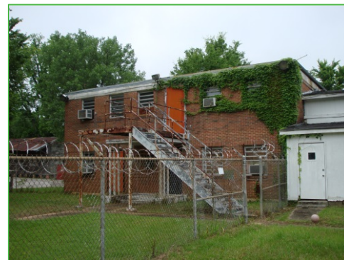
Figure 1. Lowndes County Jail is one site considered for a future transit stop along the Trail.
