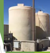
High Strength Waste Tanks
