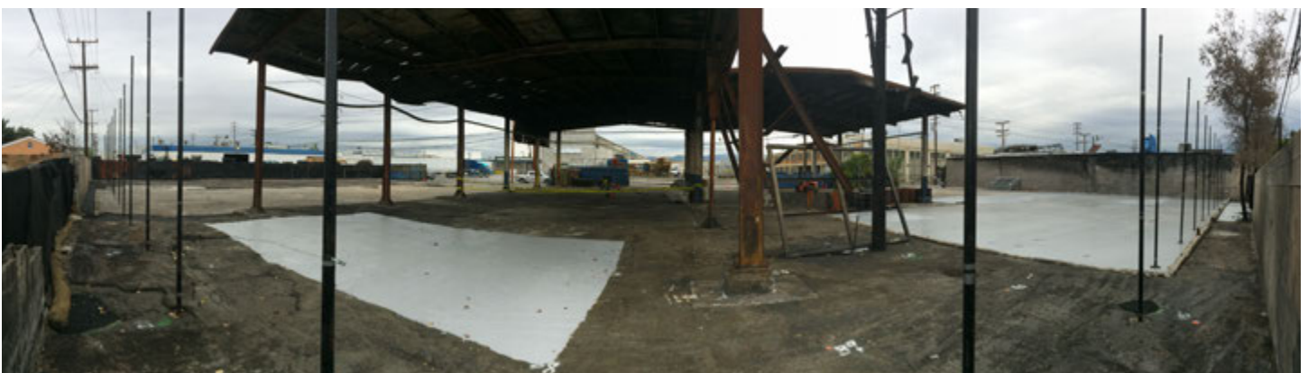
Example of area where epoxy coating has been applied
