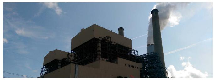
Figure 4: Photo of the plumes from CRPP Units 4 and 5 merging upon exit from the shared stack.
