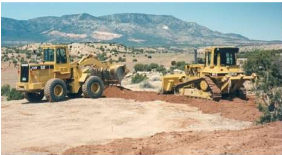
NAMLRP reclamation site NA-0804 at Lookout Point Incline Mine. This photo shows a loader hauling Class A cover and a bulldozer placing it on a reclaimed waste pile. Photo courtesy NAMLRP.
