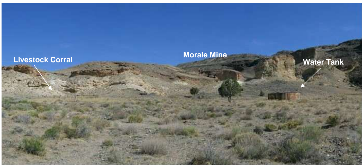
Photo showing the reclaimed Morale Mine with a water tank and livestock corral in close proximity. Photo courtesy TerraSpectra Geomatics (photo taken May 2006).
