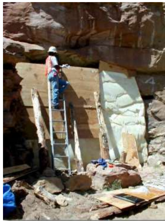
Figure 10. Polyurethane Foam (PUF) Closure on an Open Portal. Photo courtesy NAMLRP.
