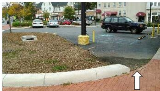
Photo 14-3. Inappropriate grading is another common design flaw in infiltration-based control practices. If a parking lot, street or other impervious surface is not properly graded towards the control or is bypassing the control, the BMP is not serving its intended purpose. In the photo above, the wet spot on the pavement indicates either poor grading in the installation or poor drainage by the control. Consider adjusting the grade. (Credit: EPA Region 5)
