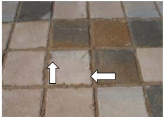
Photo 14-6. Fine mud and silt in between permeable pavers hindering rapid infiltration. (Credit: Bill Hunt, NCSU)
