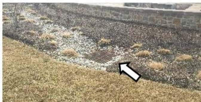
Photo 14-4. If the outlet is set too low, then stormwater will not pond and very little water will infiltrate, as it is designed to do. (Credit: John Kosco, Tetra Tech)
