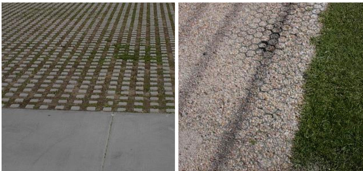
Exhibit 14-8. Grid Pavers—Concrete (left) and Plastic (right) (Credit: Tetra Tech)
