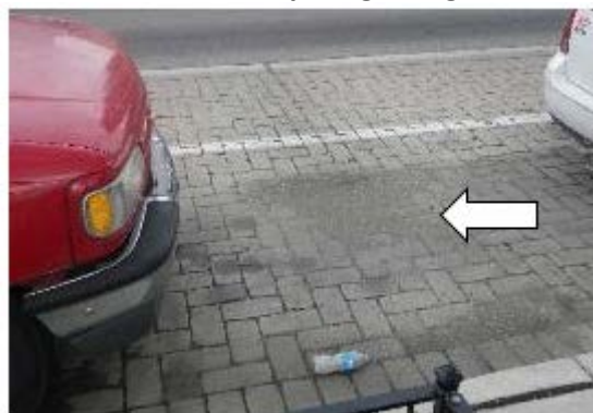
Photo 14-8. Visible silt on the permeable pavement surface, indicates that water is collecting before infiltrating. Maintenance, such as sweeping or vacuuming is needed. (Credit: EPA Region 5)
