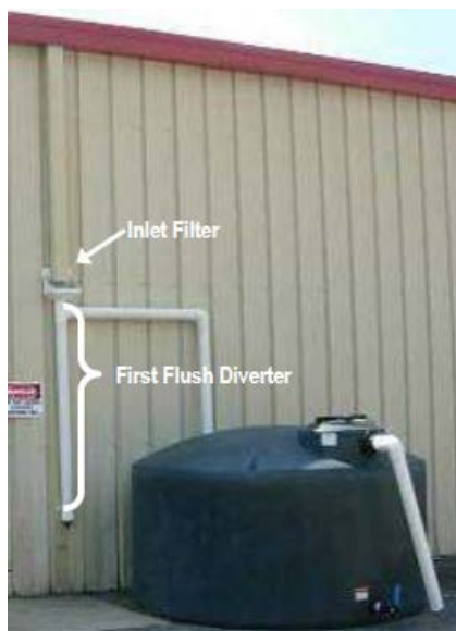
Exhibit 14-10. First Flush Diverter (Credit: NCSU BAE)
