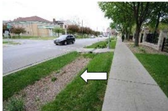
Photo 14-2. Bioswale treated with herbicide accidentally. Vegetation is sparse, which may allow erosion. Consider reseeding or replanting and providing adequate signage in English and Spanish to ensure the practice is not continually treated with herbicide. (Credit: EPA Region 5)
