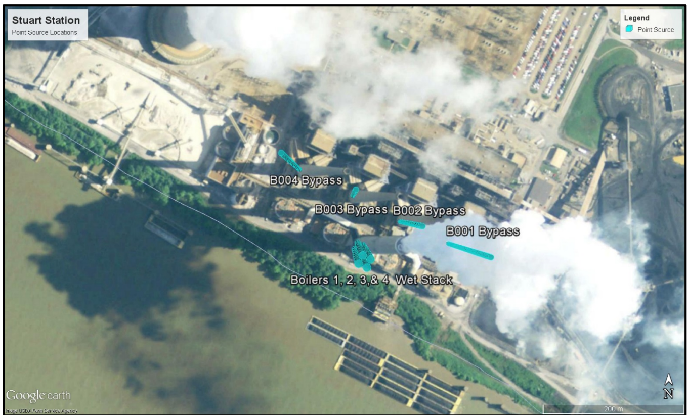
Figure 1. Stuart Station Stack Configuration
