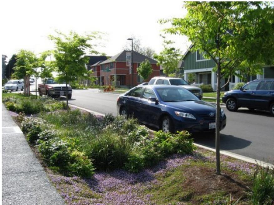
Street side swale and pervious concrete sidewalk, Seattle, WA
