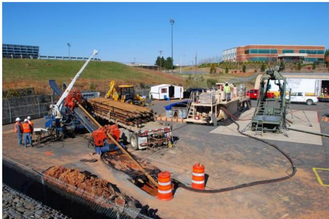
*Typical well drilling equipment setup*
