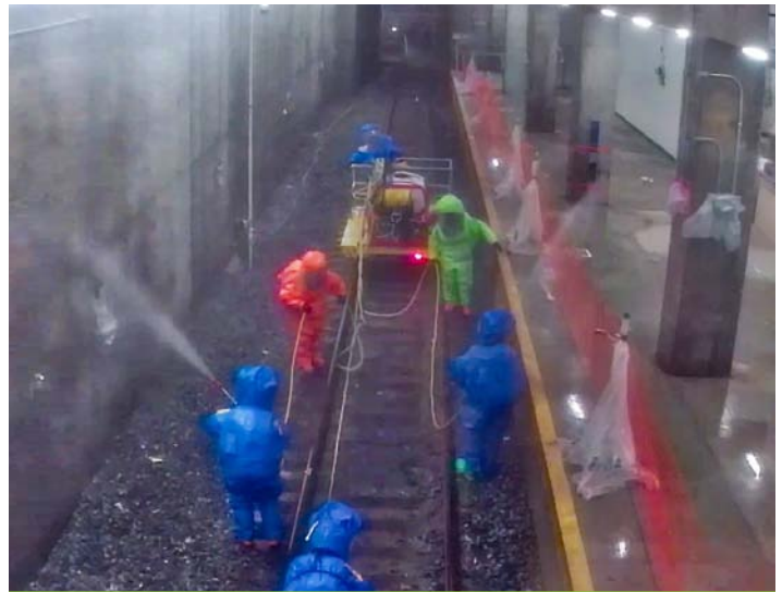
Region 3, CMAD and NHSRC complete spray decontamination of the tunnel
