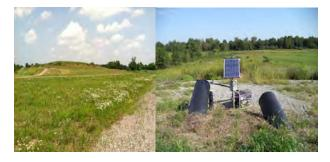
The CAMU is monitored by a remote system which alerts the caretaker of excess leachate (liquid) pools in the collection system.
