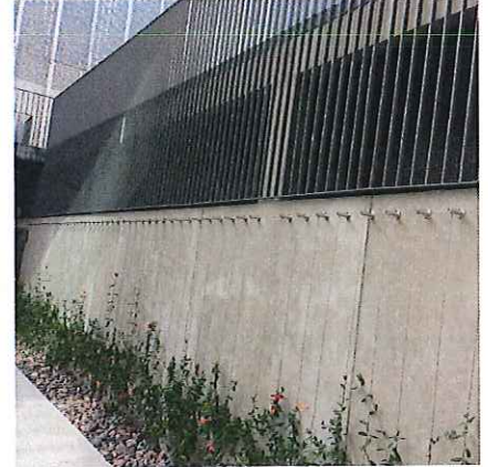
Energy Recovery Ventilation to Green Space providing cool in summer & heat in winter
