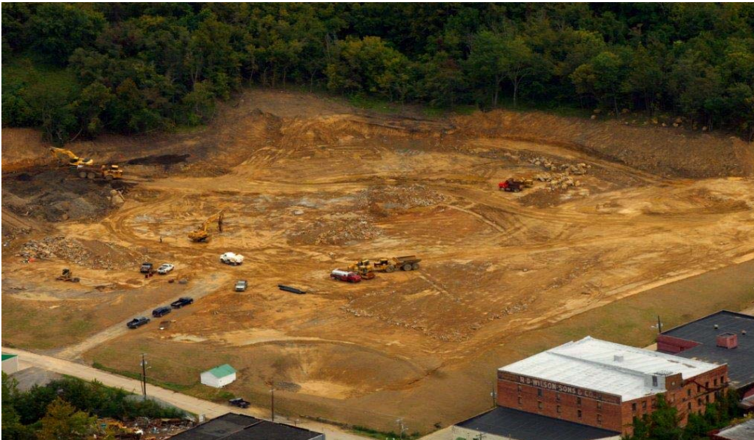
Site before construction
