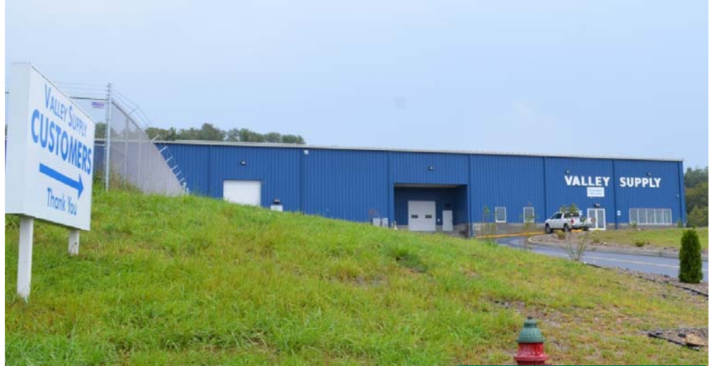
Site after construction
