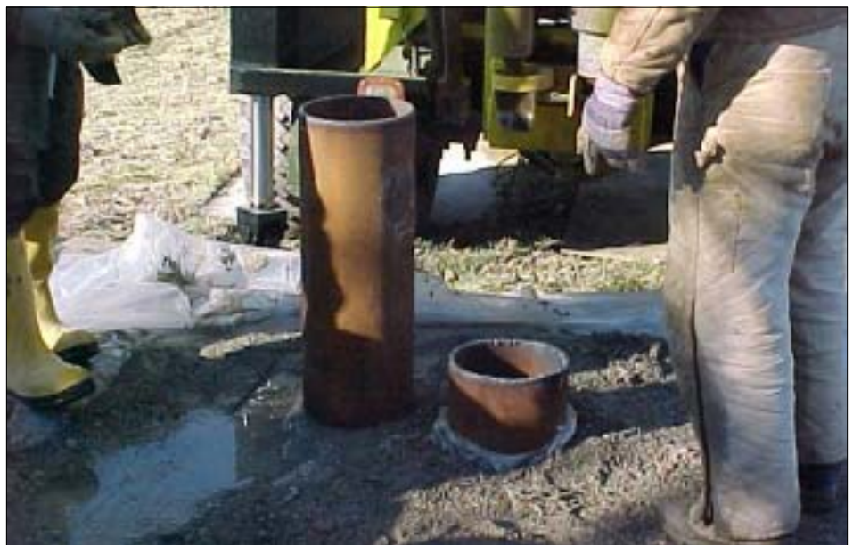
Vernay's contractors install a second pumping well on the property to pump ground water to the surface for treatment to remove contaminants.
