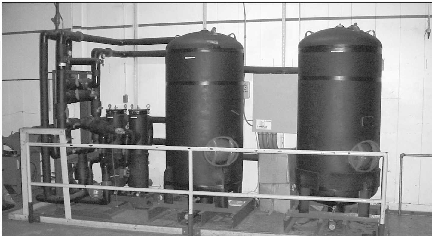
Contaminated ground water brought to the surface by the capture wells is treated using carbon filtration and is then discharged into the sanitary sewer.
