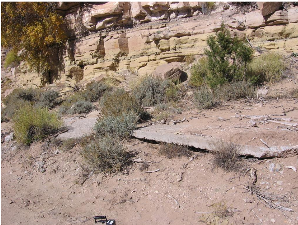
Photo 6. Mine site #508 concretepads
