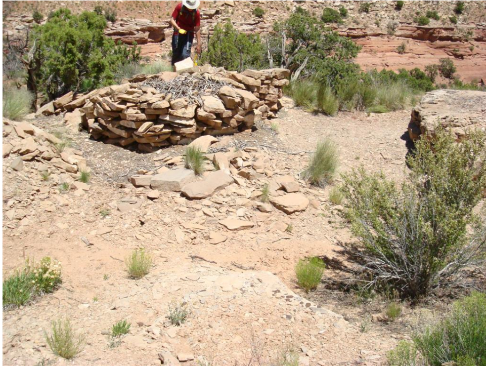
Photo 9. East Workings site #185, capped area
