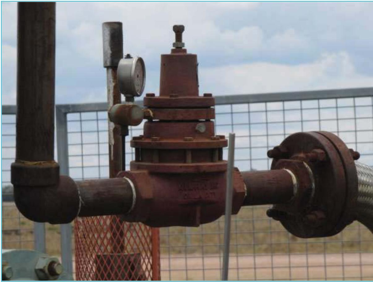
**Figure 5.2. Pressure regular that was a common source of CH<sub>4</sub> leakage.**
