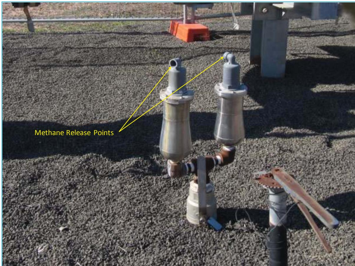
**Figure 4.7. Methane emission sources on a water gathering line.**
