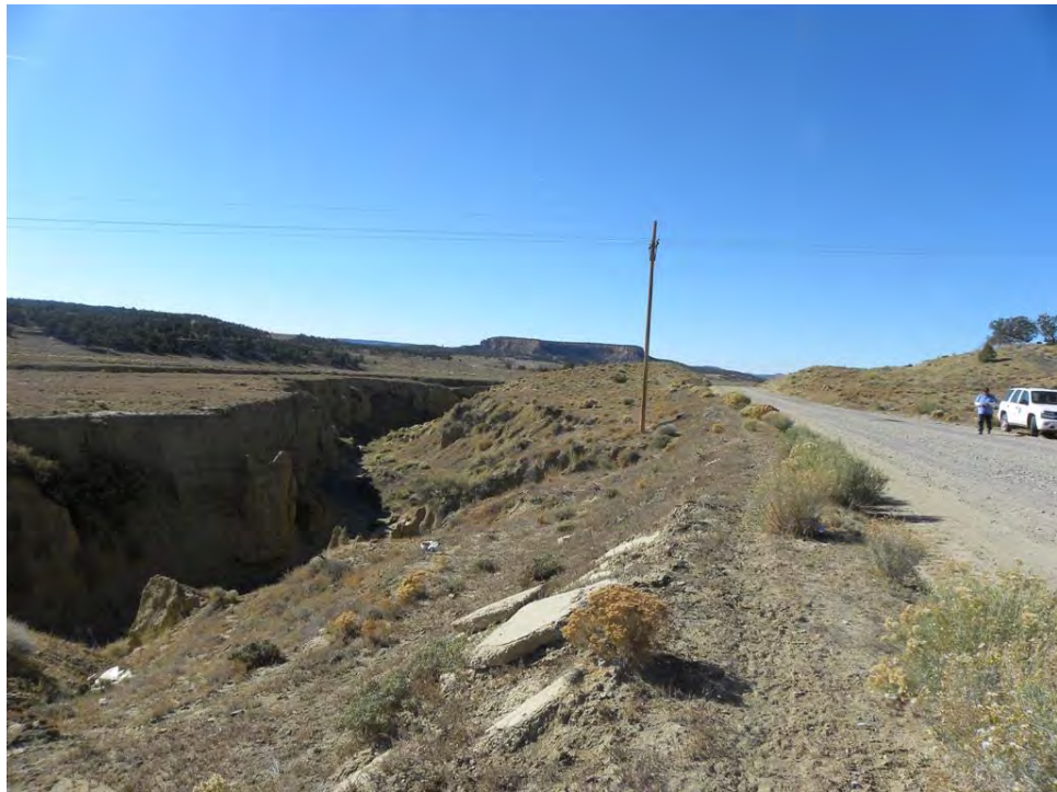
Photo 4. NE Church Rock 1-East drainage to arroyo
