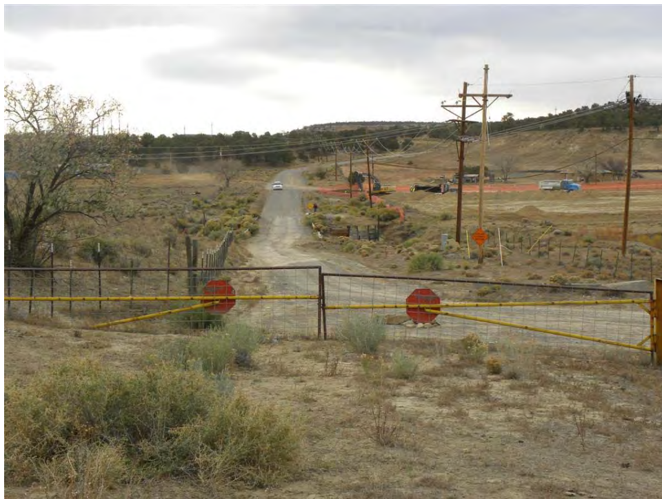
Photo 2. Entrance to NE Church Rock 1 gate and bend in road
