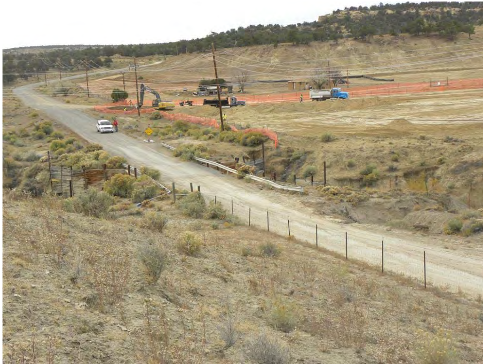
Photo 1. Road and bridge separating NE Church Rock and NE Church Rock 1
