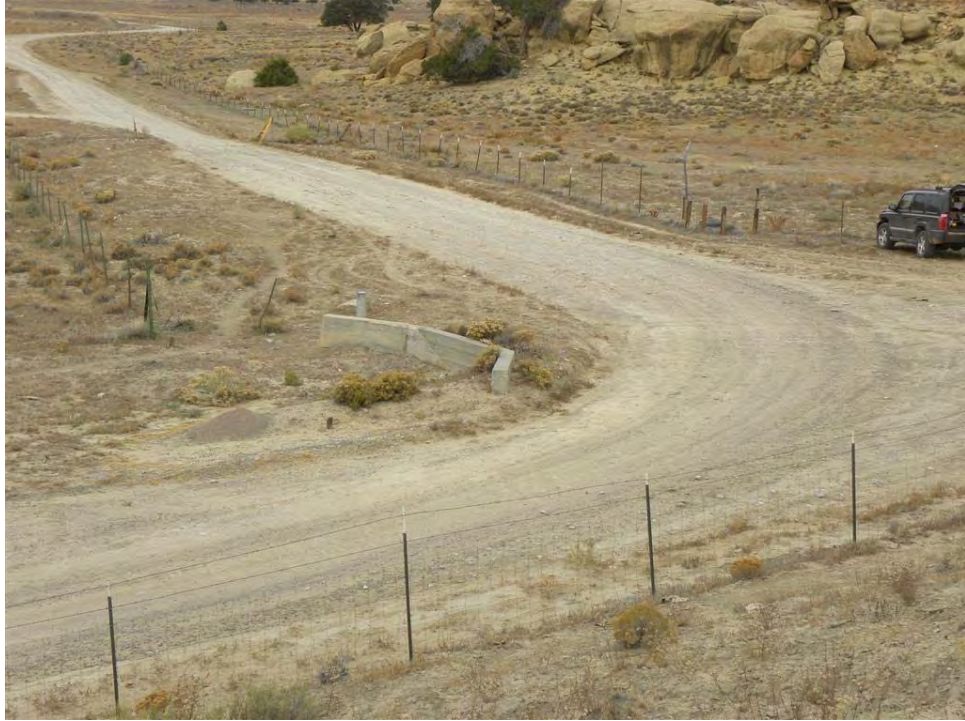
Photo 3. Bend in road and culvert outfall
