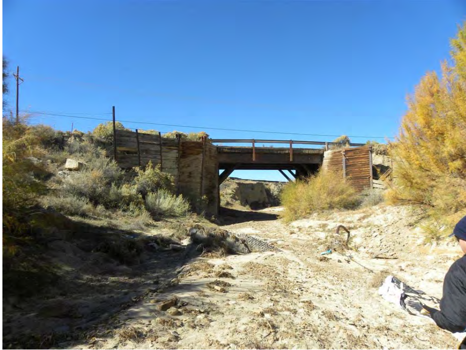
Photo 9. Bridge crossing arroyo between NE Church Rock and NE Church Rock 1
