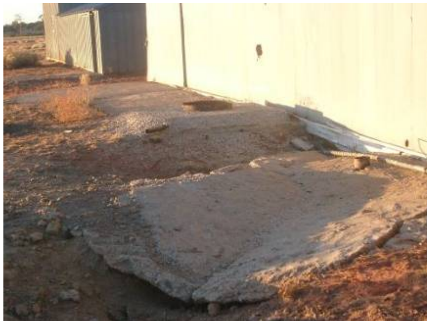
Photo 8. Concrete pads on south side of grey buildings
