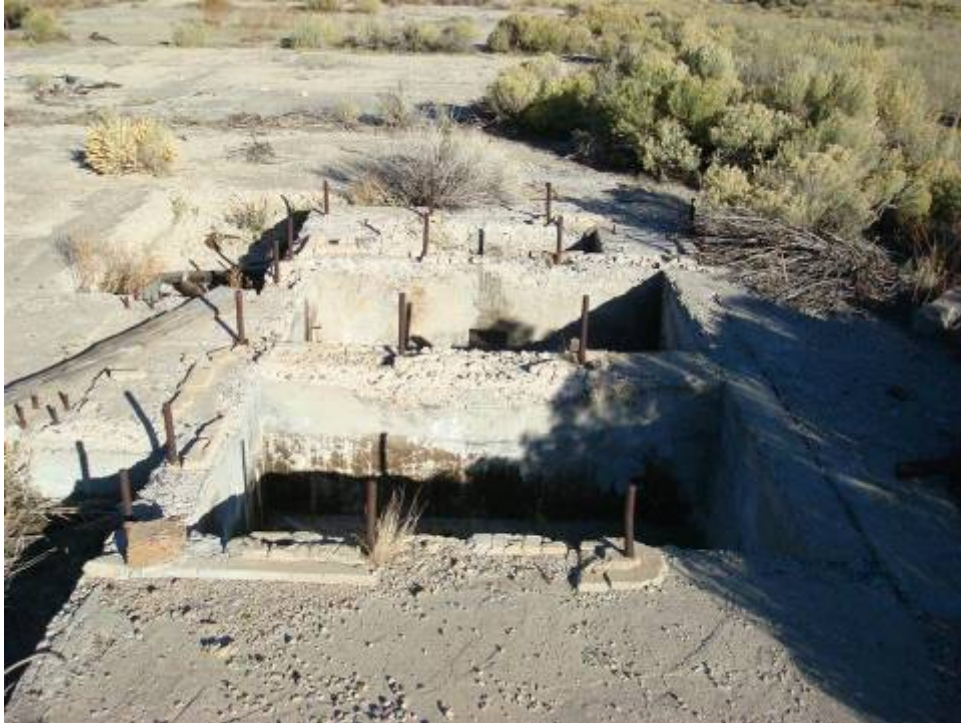
Photo 3. Black Jack No. 1 Mine site, clarifiers or vaults.
