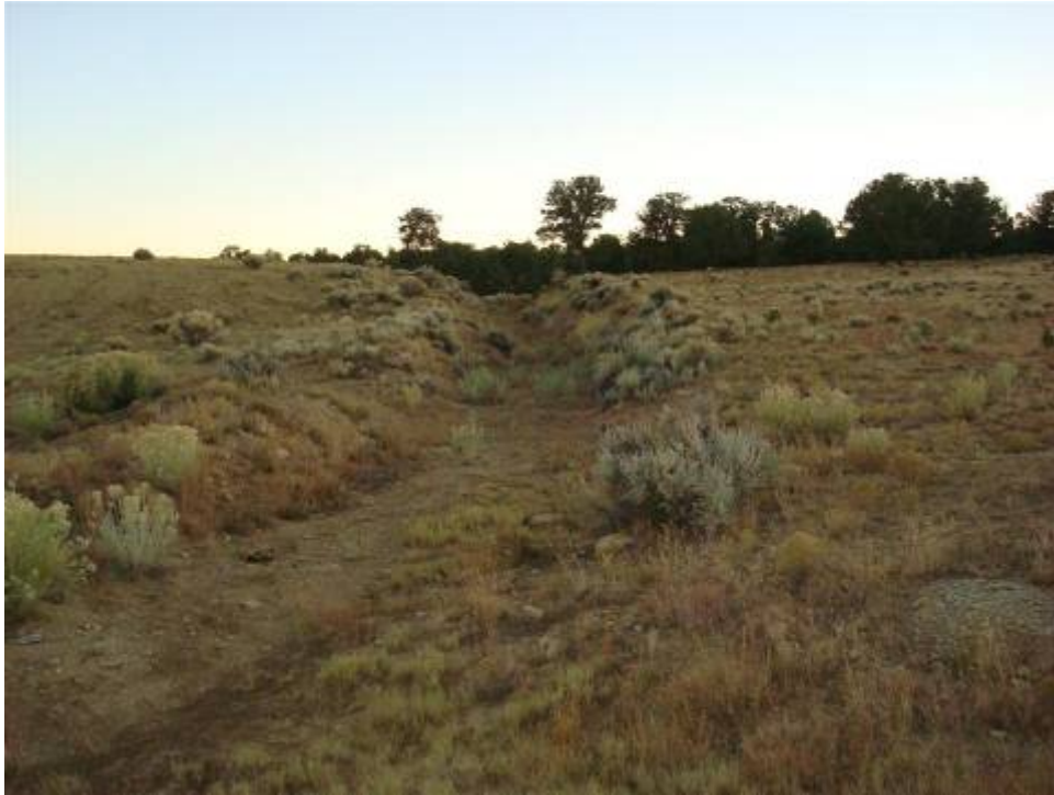
Photo 3. Ruby No. 3 Mine site, erosion of southern portion of mine
