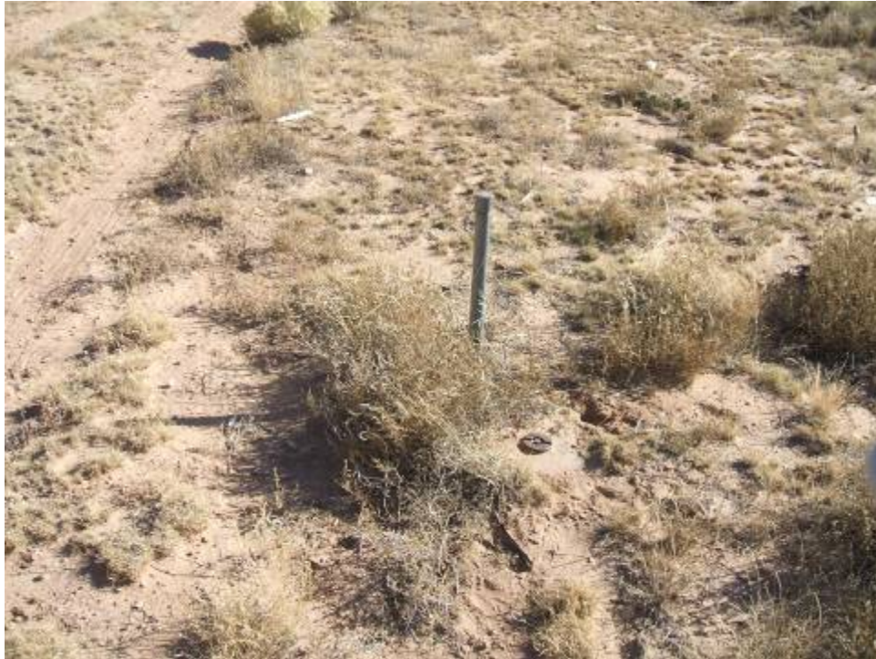
Photo 5. Haystack mine site 1039, water pipe, towards the south
