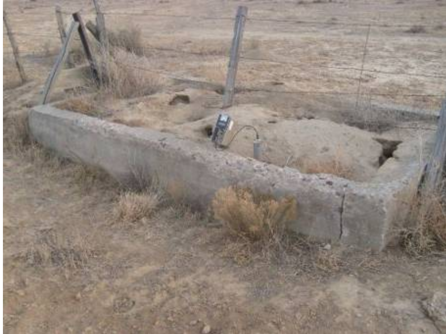
Photo 9. Concrete vault along south fence
