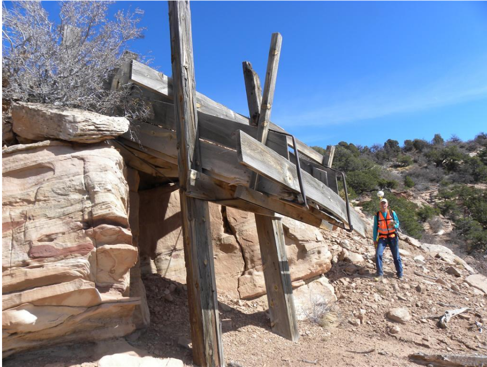
Photo 3. Wood framed chute
