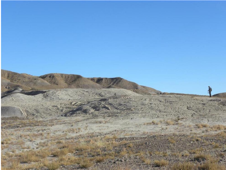
Photo 3. Charles Huskon No. 9 mine site, reclamation cap
